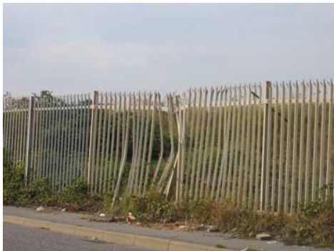
Old style industrial palisade fencing
